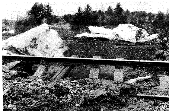
Figure 3: Damaged railroad track caused by ice cakes and high water from the Ammonoosuc River, New Hampshire.
